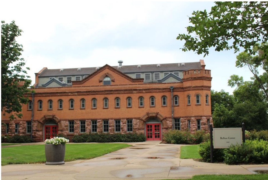
3. Armory/Gymnasium (Old), south elevation (camera looking north)
