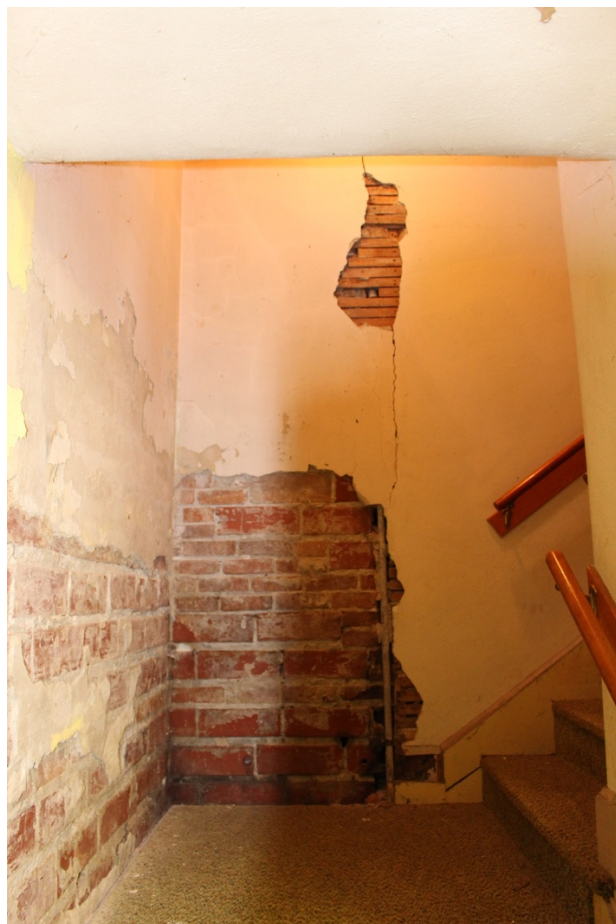
Areas of cracked and missing plaster in stairwell to basement
