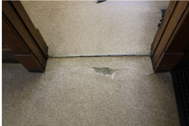
Cracked and chipped flooring
