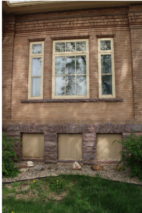
Grouping of windows on main level includes large center window flanked by narrower windows; storm windows have narrow muntins; criss-cross muntins of original interior windows are visible through the storm windows; basement windows are covered with a composite vertical siding material
