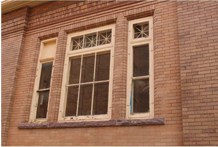
Example of deteriorated storm windows showing need for paint and repair
