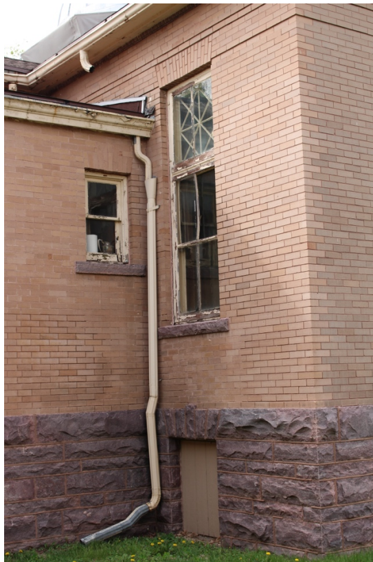
Downspout allows for water the enter building along the foundation
