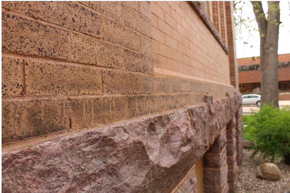
Exterior wall (north) showing quartzite stone base, speckled brick and solid-colored brick
