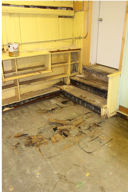
Damage to floor at south entrance
