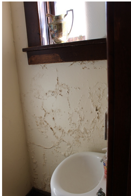
Plaster damage in restroom
